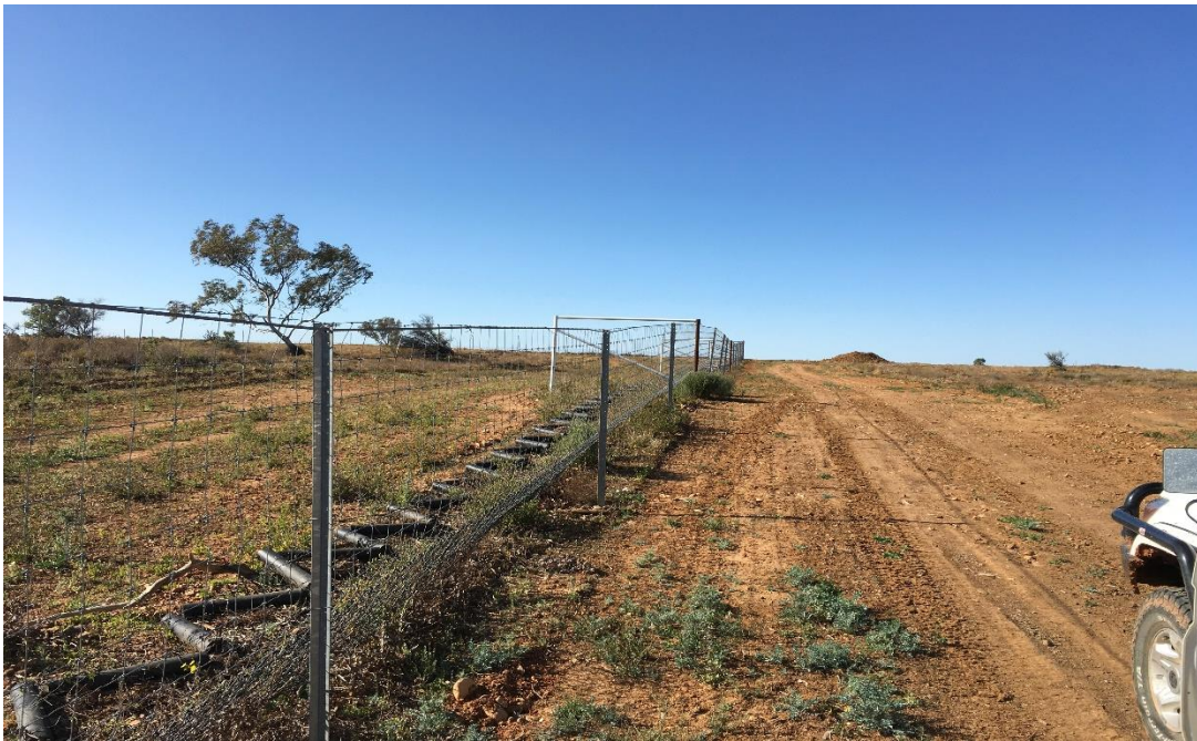
A section of fence that has recently been repaired together with flood gate
